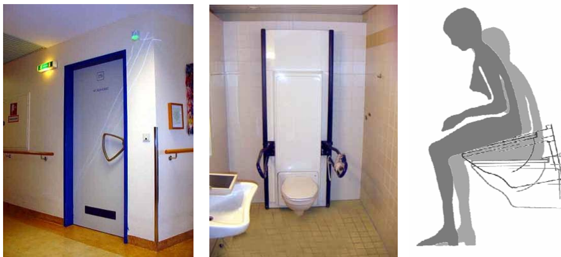
Figure 1: Toilet room at day care centre for MS patients for the FRR real life test Dec 2004 - Feb 2005: door with door handle (left), height and tilt adjustable toilet system (middle and right).
